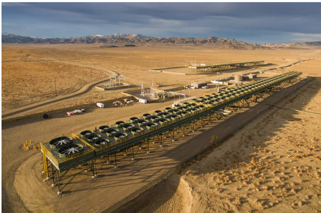
Figure 2 - Typical Geothermal Facility (Note: top of air coolers 40' above grade)
